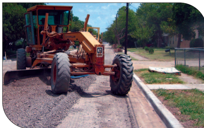
Initial shaping and grading.
