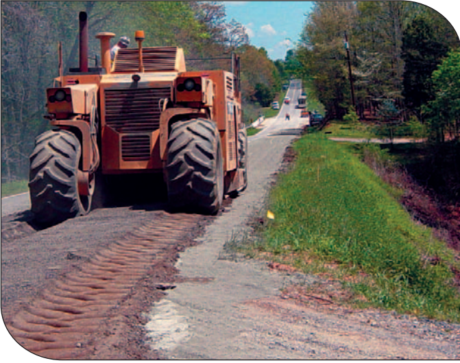
Recycling old asphalt pavement using FDR.
